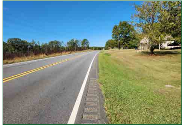
Looking west at the access point on AL Hwy 77.
