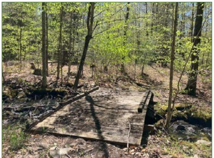
An ATV bridge providing access through the tract.
